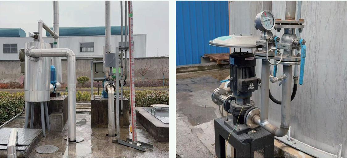
COSMOS Ma'anshan Deploys Reclaimed Water Pumps and Collection Sumps in Tank Farm
